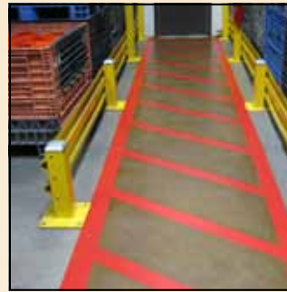
Fire Exit Markings
